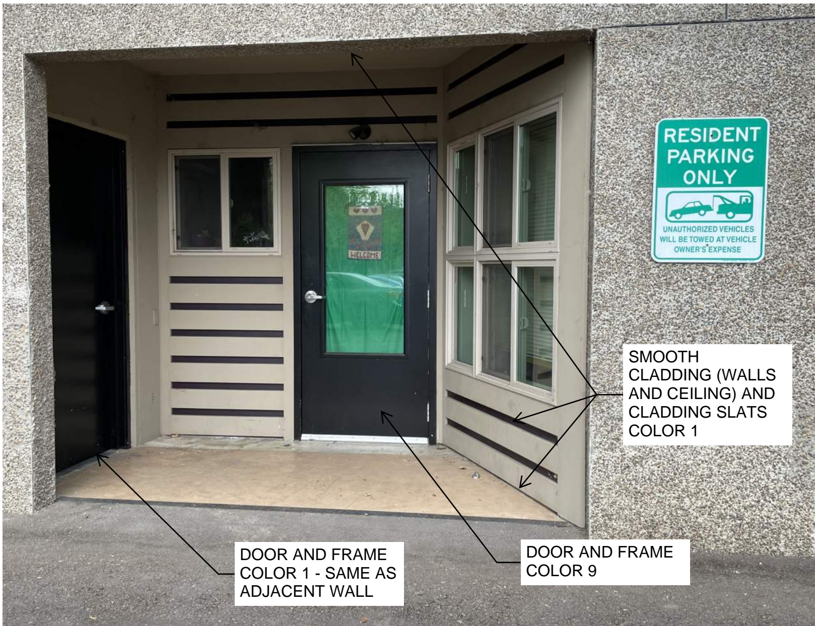
EXTERIOR DOORS AT EAST WALL OF SOUTHWEST WING - SEE 1/A214
