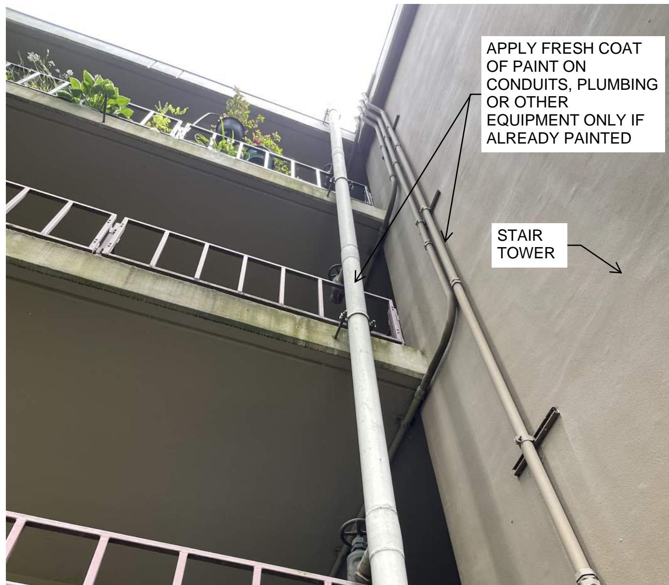
PAINT AT ELECTRICAL CONDUITS AND FIRE RISER BY STAIR TOWER
