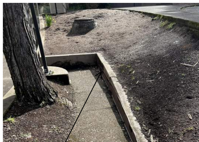
CLEAN DEBRIS AND APPLY NEW CAULK AT WALL / SIDEWALK TRANSITION JOINT PER MANUFACTURER'S INSTRUCTIONS.
