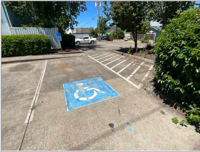
OVERVIEW OF ACCESSIBLE PARKING AREA
