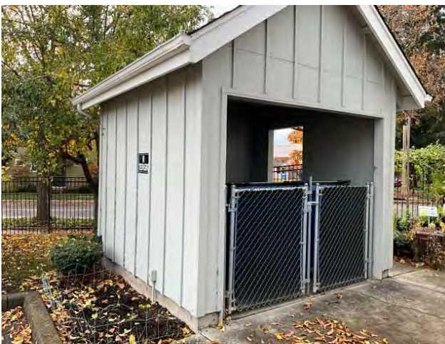
23 - GARBAGE RECYCLING STRUCTURE
